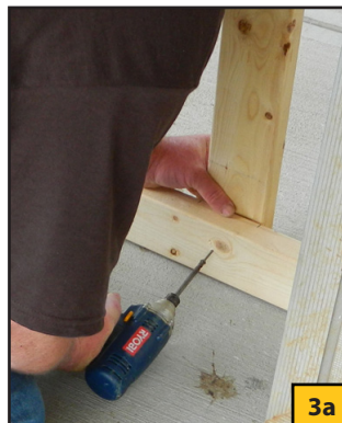
Three-inch deck screws secure the frame uprights to the base assembly.
