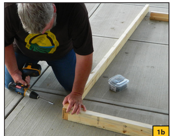
A couple of deck screws per corner secure the base assembly 2x4s.
