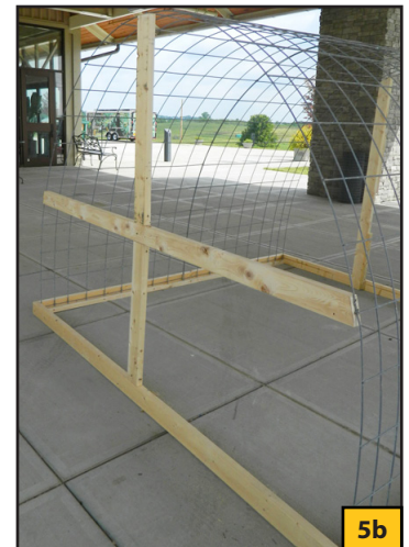
Cut the uprights to length, and secure them to the base, the crossbar, and the hoop.
