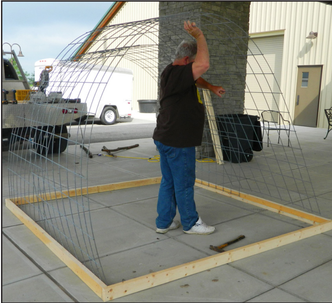
When bent, the 16-foot long cattle panels form a hoop approximately 6 feet in height.
