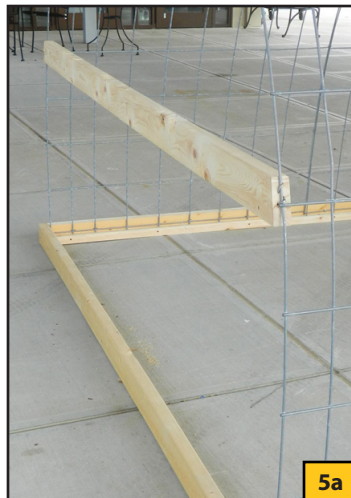
Cut the crossbar to length, and attach it to the hoop with fence staples.
